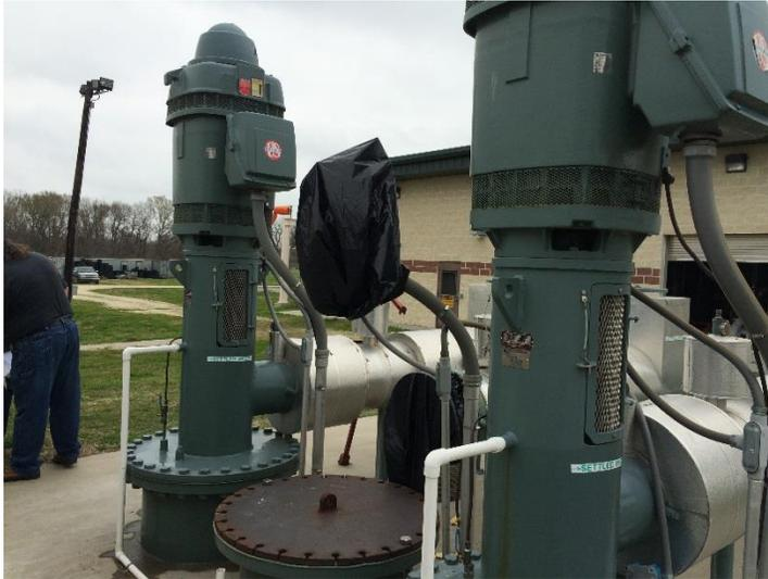
The filter feed pumps provide feed water to the membrane filters in the Filter Building. The water treatment plant utilizes pressure-driven ultrafiltration membrane filters. Thus, the filter feed pumps provide pressure for the membrane filtration system. Three (3) vertical turbine pumps are used to provide pressurized water for the membrane filters. The pumps are installed with VFDs which are controlled by the membrane filtration control system and connected to the SCADA system.
