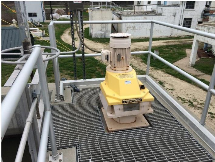
Currently, there are no operational issues with the raw water splitter box and rapid mixers. However, one of the rapid mixers is showing evidence of a bent shaft.
