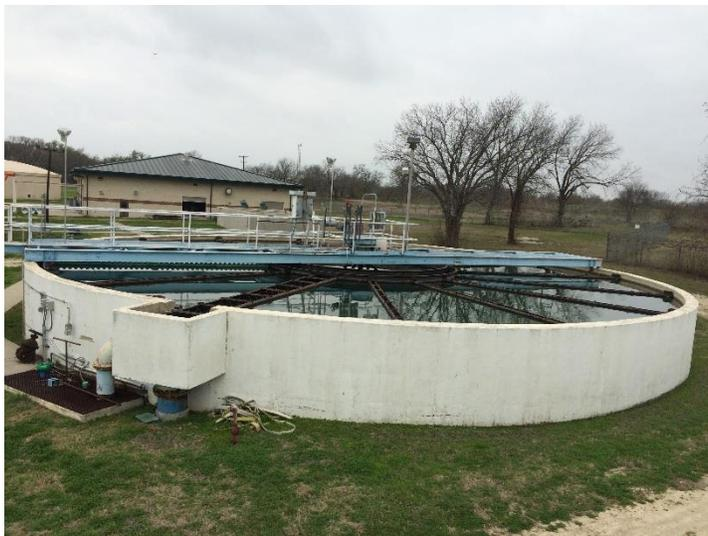
The mixer in Clarifier No. 2 is not operational. Without mixing energy in the reaction-flocculation zone, more coagulant is necessary. The operators are currently feeding more coagulant yet are still seeing higher turbidities in the settled water as
