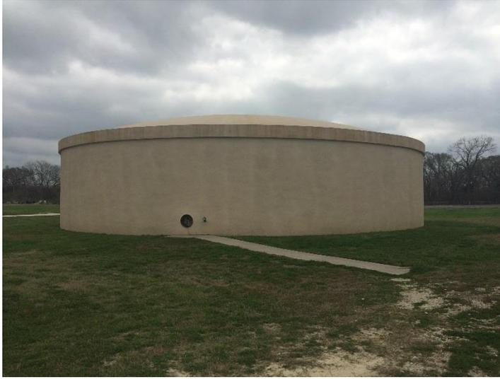
Water is removed from the clearwell by the high service pumps based on system demands or by a backwash pump based on the need to backwash a filter. No special controls are required for the clearwell. The SCADA system indicates the level of the tank for the operator's information and use.
