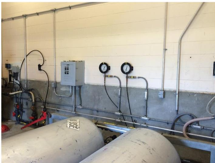
Chlorine can be added prior to the clarifier at the splitter box, at the filter feed wet well, and prior to the clearwell in the two effluent lines from the membrane filters.
