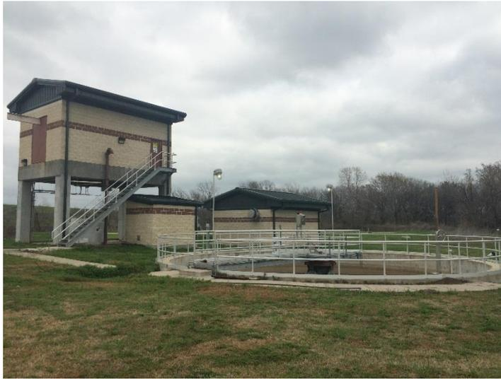
The sludge thickener receives drain water from the reclaim ponds and the filter feed wet well, decant water from the centrifuge, sludge blowdown from the two clarifiers, and the initial sludge/water mixture when a clarifier is drained.
